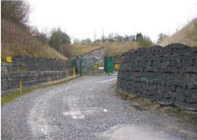
The main entrance to Milldam Mine in happier times (Image: Mindat)
