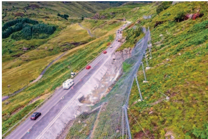
This is the main working site on the A83, at a place called Rest and be Thankful, where recent heavy rainfall has led to further landslips despite the work going on to alleviate them in the long term. (Image: Bear plc)
