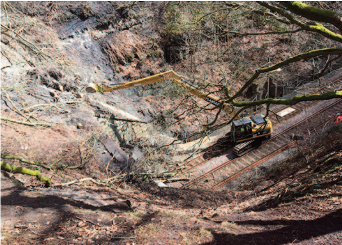
It's almost a case of 'spot the railway' - this is the scene at the mouth of Baildon Tunnel on the Leeds-Ilkley line. (Image: Network Rail)
