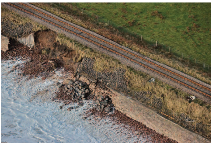
Scotland's Far North Line runs along a low seawall between Brora and Helmsdale, even getting to this remote spot with suitable equipment isn't easy. (Image: Network Rail)
