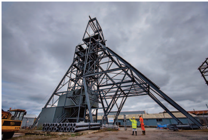
The headgear at South Crofty Mine, where work underground is moving ahead with the help of the National Wealth Fund.
