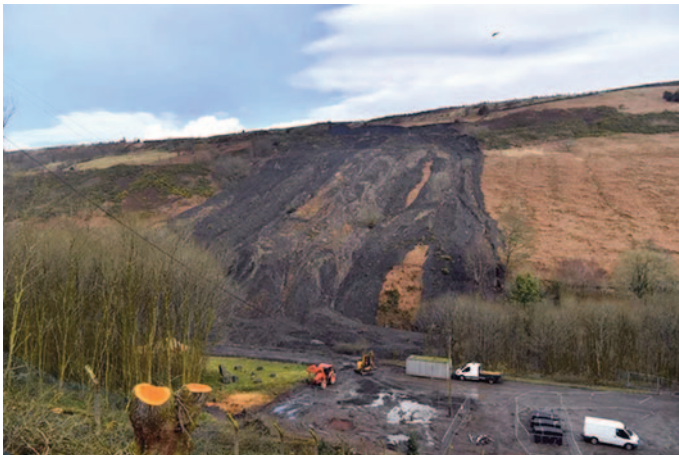
The Tylorstown slip of 2020 involved an estimated 60 000 tonnes of material. (Image: WalesOnline)
