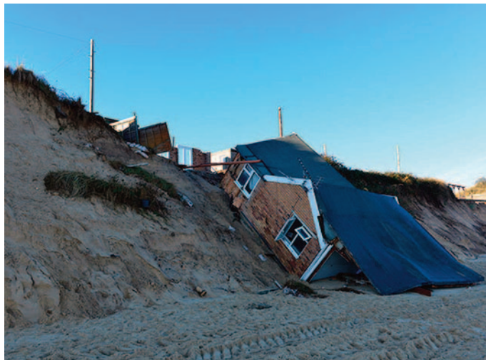
Flashback to storm surge in December 2013, this was the scene at Hemsby as a home slips over the edge in a surprisingly good state of repair. (Image: BGS)
