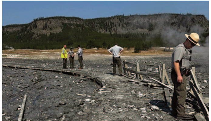
The scene as National Park Staff assess the damage to Biscuit Basin boardwalks after a hydrothermal explosion (Image: National Park Service)
