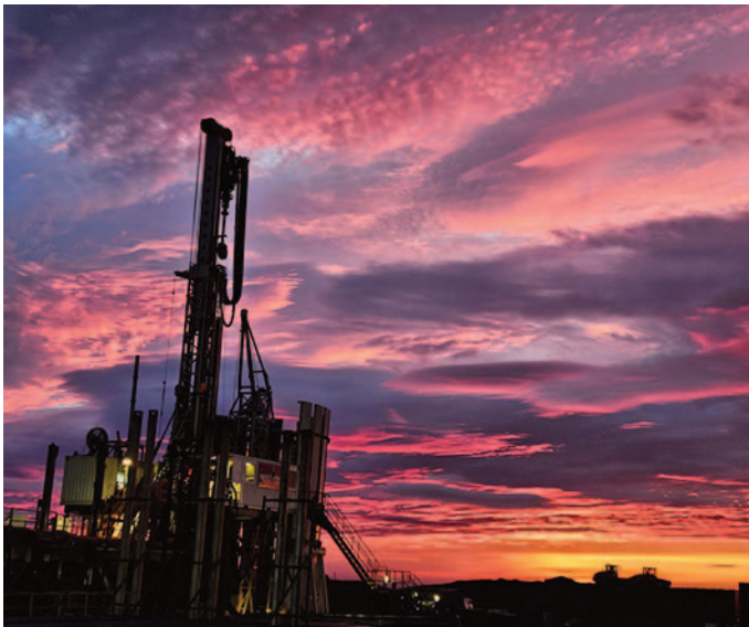
A recent image of Rig 50 at the Woodsmith Mine site near Whitby. (Image: Callum Fitzpatrick via Facebook)
