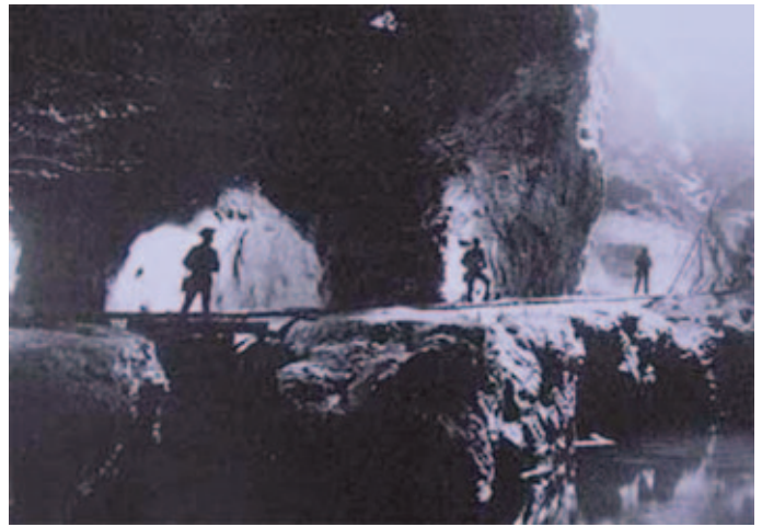
Inside Garth Iron Mine, an image taken when the mine was working in the nineteenth century.
