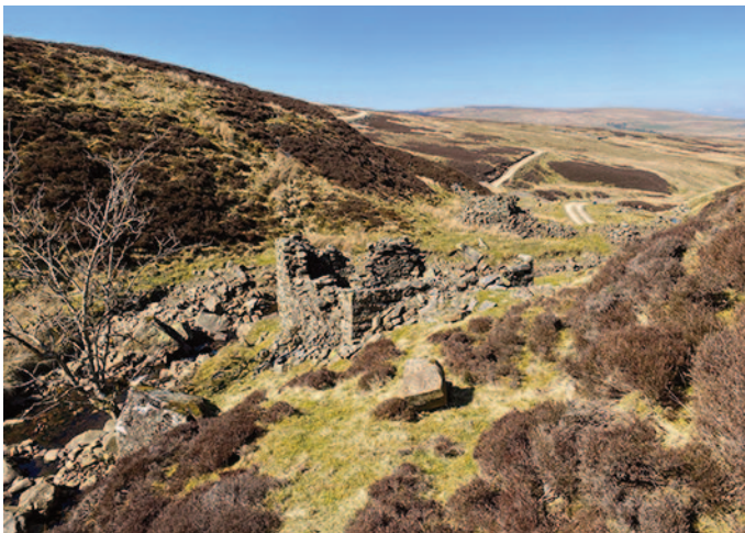
The derelict mine shop and an adjacent mountain ash tree on the reclaimed site of Smittergill Mine.
