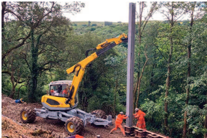
Inserting a length of pile at the Hague Bar site. (Image: Network Rail)
