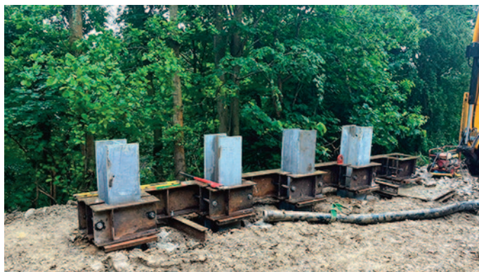
The pile and wall solution in progress of being built at Hague Bar. (Image: Network Rail)
