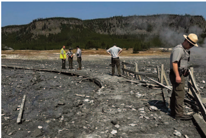
The scene as National Park Staff assess the damage to Biscuit Basin boardwalks after a hydrothermal explosion (Image: National Park Service)
